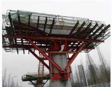
Overpass box girder formwork
