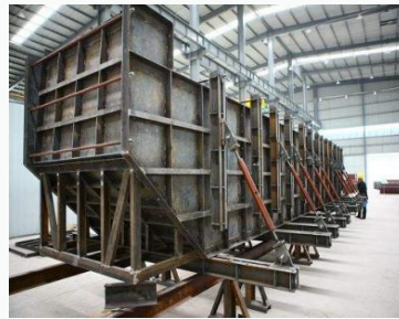
Overpass bent cap formwork
