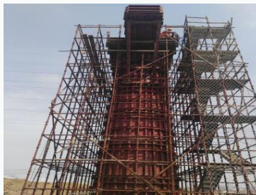
Overpass column formwork
