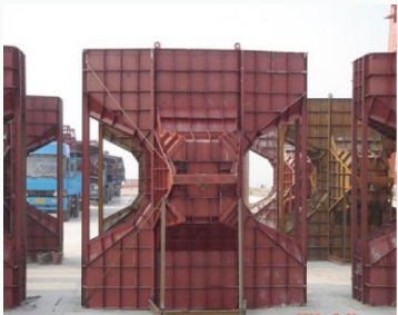
I-beam formwork
